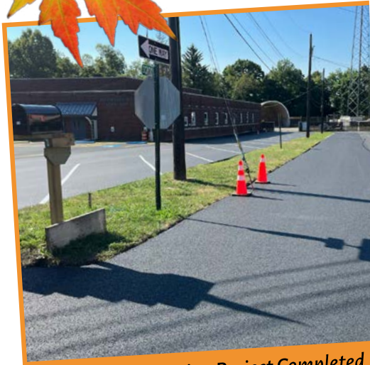
School Court Paving Project Completed
