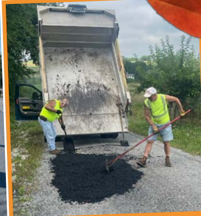
Joe & Donnie completing patch work all over the Township Roads on a hot day in August
